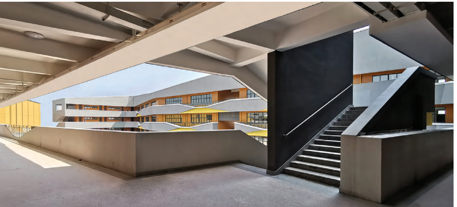
Corridor space. Photo: © Gao Pan
